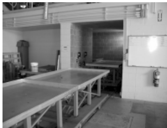
Conveyor cart with system used to carry targets through the accelerator beam.
